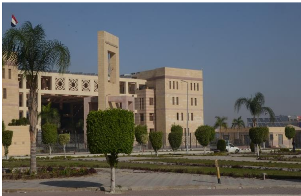
Figure 24: NUCA Building in Sheikh Zayed with Solar Panels Installed on its Roof (Farouh, 2016)
