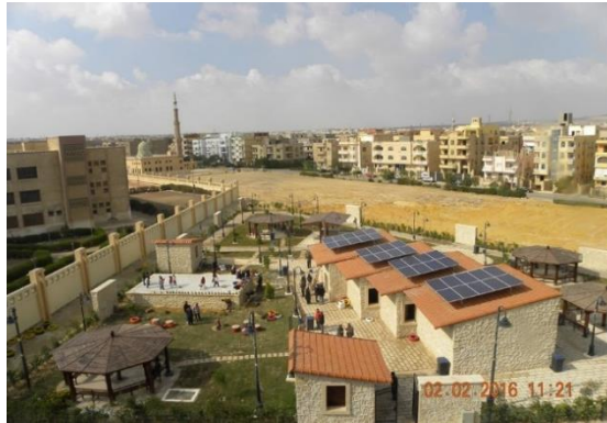
Figure 28: Showing the Environmental Garden with the Solar Panels Installed on the Roof (Farouh, n.d)
