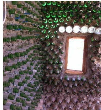
Figure 15: Glass House Built by the Community out of Reused Glass Bottles
