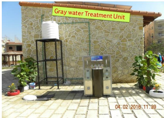
Figure 30: Showing the Interactive Grey Water Treatment Unit in the Environmental Garden (Farouh, n.d)
