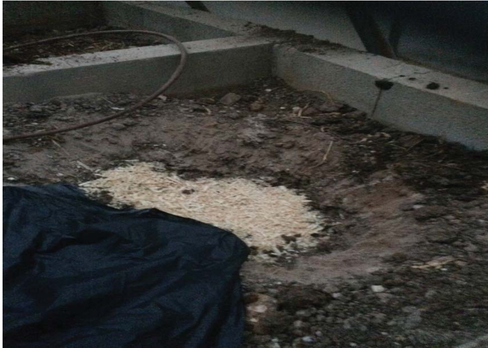
Spreading raw materials at the trenches
